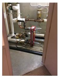
Photograph 22: Plate to Plate Exchanger.
