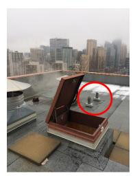
Photograph 17: Tieback Anchors.
