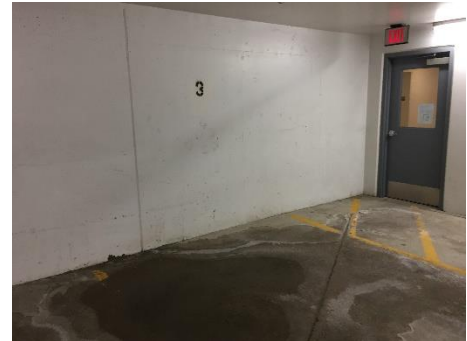
Photograph 2: Painting Finishes and Doors
